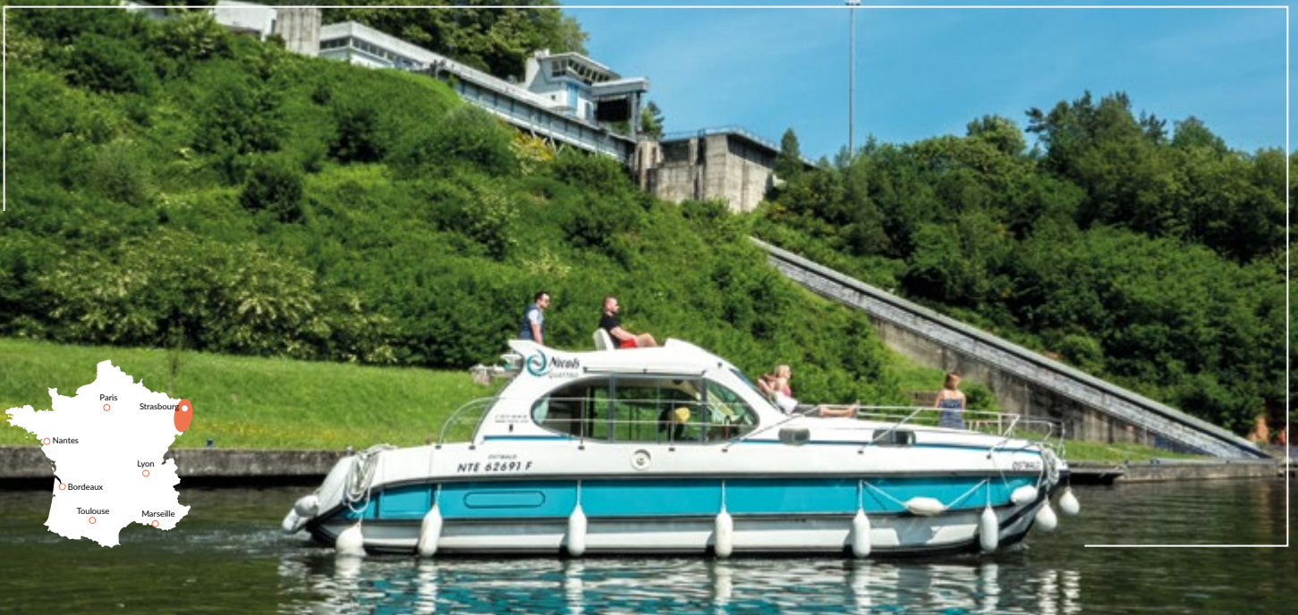
ARZVILLER - Inclined plane
