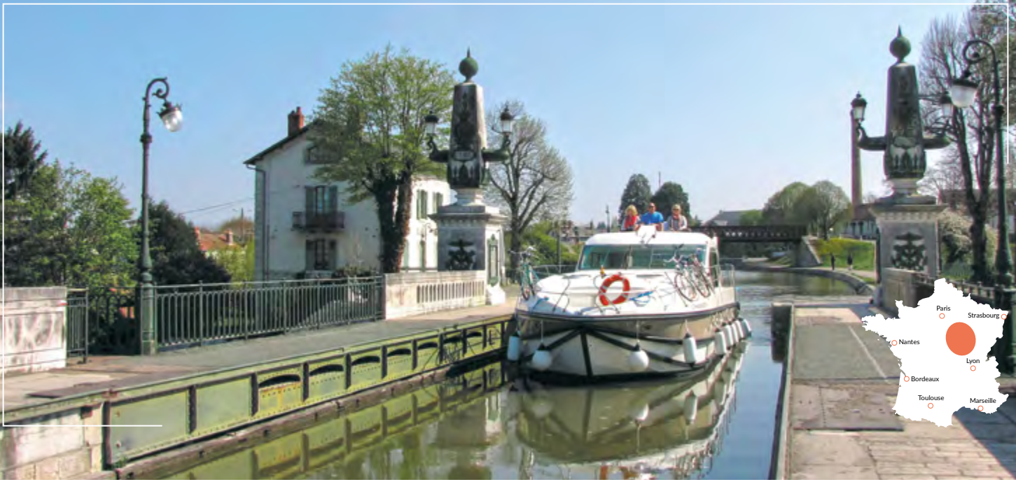
BRIARE - Canal bridge
